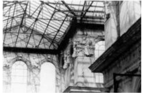
Rebuilding the destroyed cathedral, Managua, Nicaragua. Photo by Anthony McInnery
